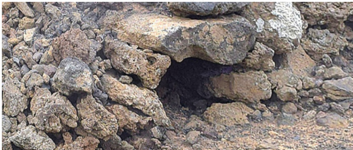
Fig.260b - One can see that the mason was anxious to reach a more or less round form of the tubus [on ground]. (Photo: Hans-Joachim Ulbrich)
